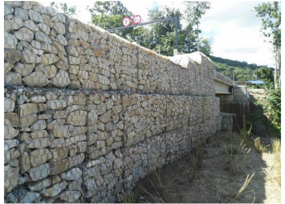
Supply of Gabion Mattress at Bentong
