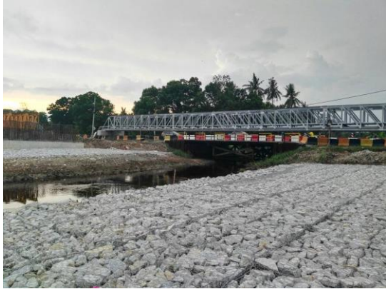
Supply of Gabion Mattress at JKR Batu Pahat
