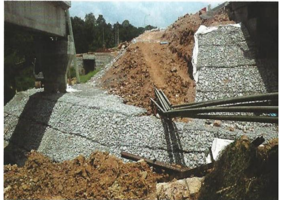
Supply of Gabion at Segamat
