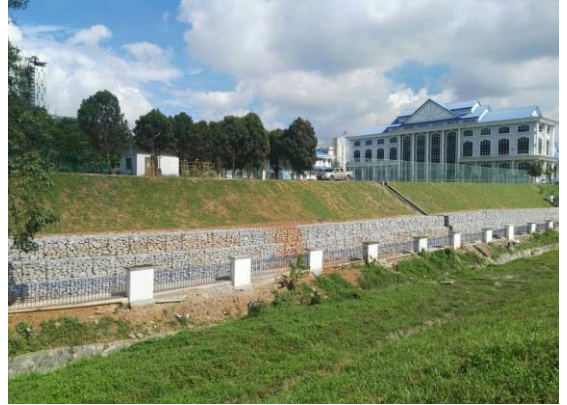
Supply of Gabion Mattress at LLM Bangi
