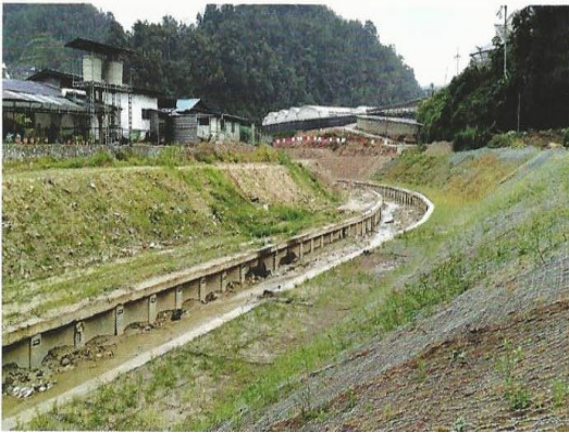
Supply of Gabion Mattress at Bertam
