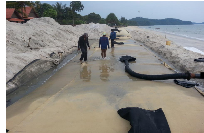
Filling of Geotube hydraulically with sand
