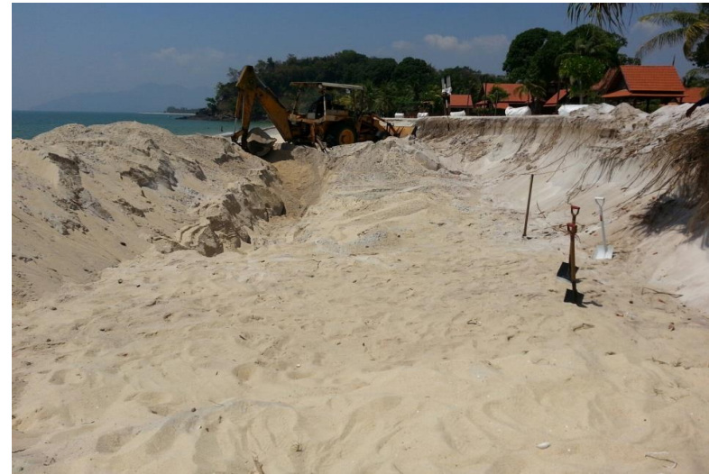
Levelling of area
