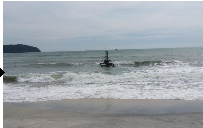
Sand pumped from seabed using submersible pump
