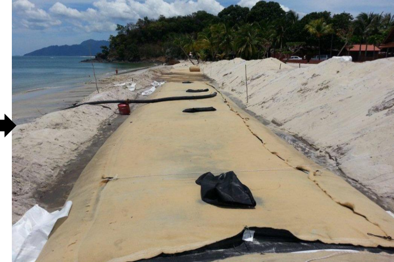
Filling Geotube
